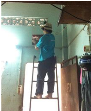
(a) Installation of Exhaust Fan through Brick Wall
